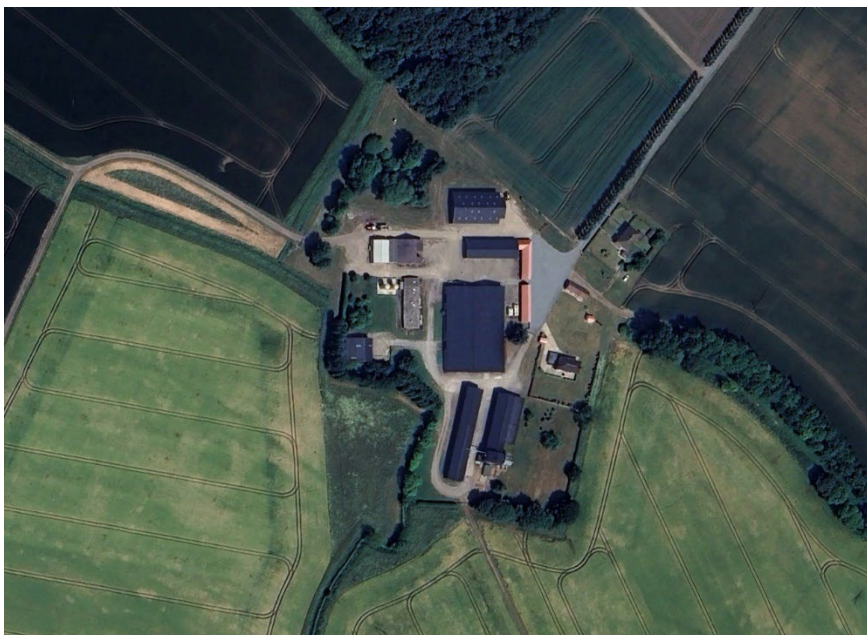
Plate 18 2023 Google Earth image of Quosquo Hall showing removal of more of the building – the last remnant of the southern range is gone.
