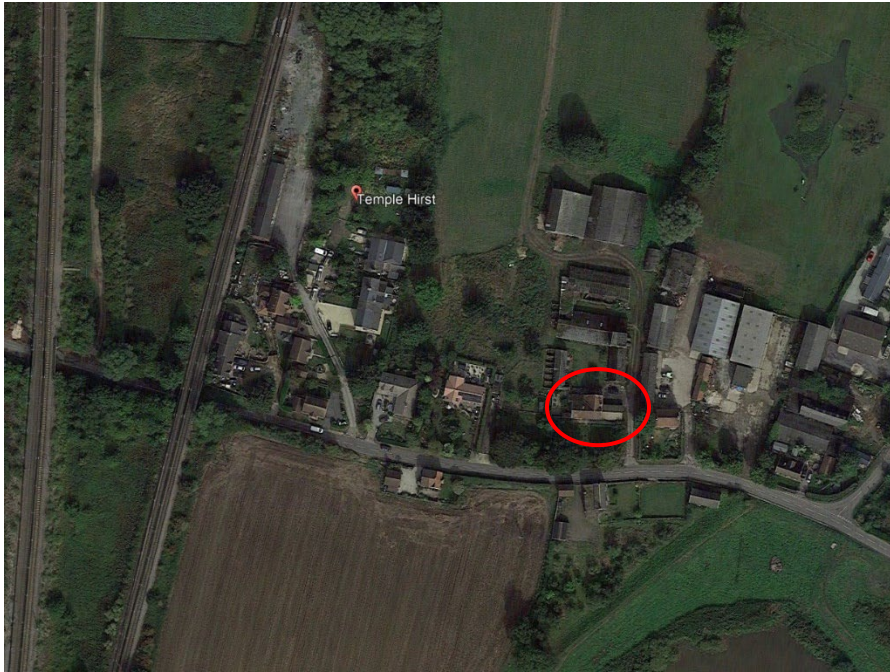
Plate 30 Aerial view of Manor Farmhouse (in red oval) illustrating large farm building to the north (Google Earth)
