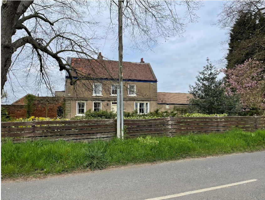
Plate 28 View of Manor Farmhouse from the road looking north
